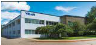
Williston, VT, U.S.A. Velan Valve Corp., Plant 3
