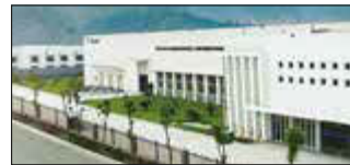
Suzhou, China Velan Valve (Suzhou) Co., Ltd.
