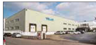
Ansan City, South Korea Velan Ltd., Plant 2
